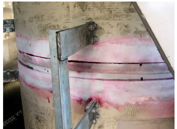
Dye penetrant test
